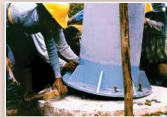
Base Plate foundation
