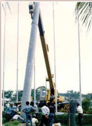
Installation by Lifting Crane
