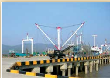
HARBOUR / JETTY STRUCTURE
