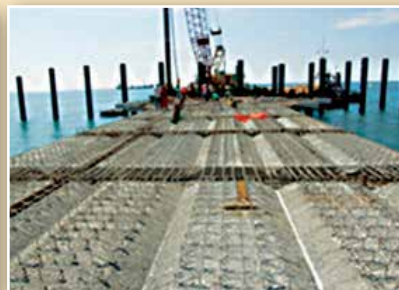
PRECAST HALF SLAB
